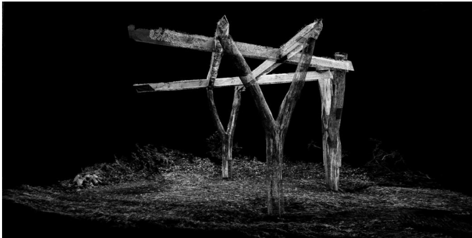
Fig. 1. Photogrammetric 3D scan of the Foundry after 'Chainsaw Choreographies'. This precise survey confirmed the accuracy of fabrication and served as a base for further development.
