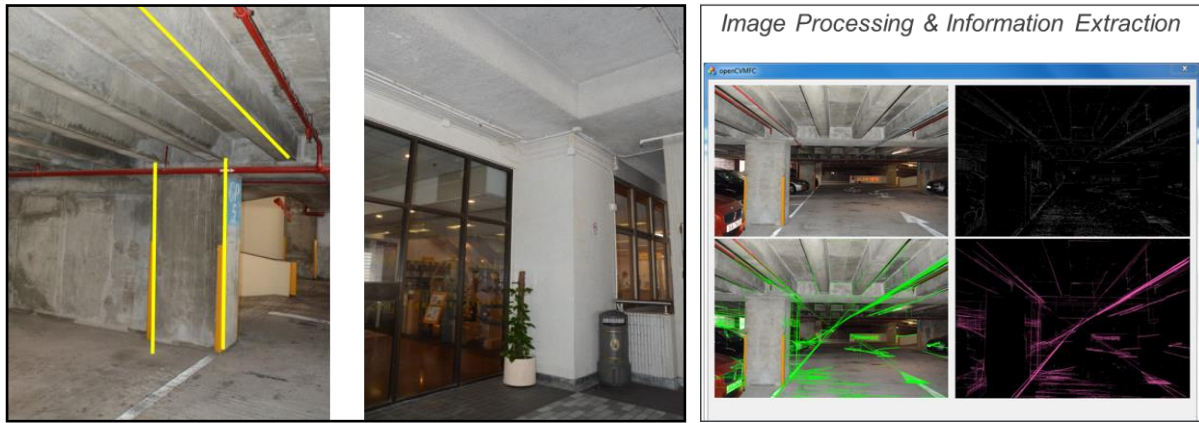
Figure 7 Structural components in a typical building (photos taken by author (left part); Image processing and information extraction using Hough Transformation (right part) (revised from Lu and Lee 2016)
