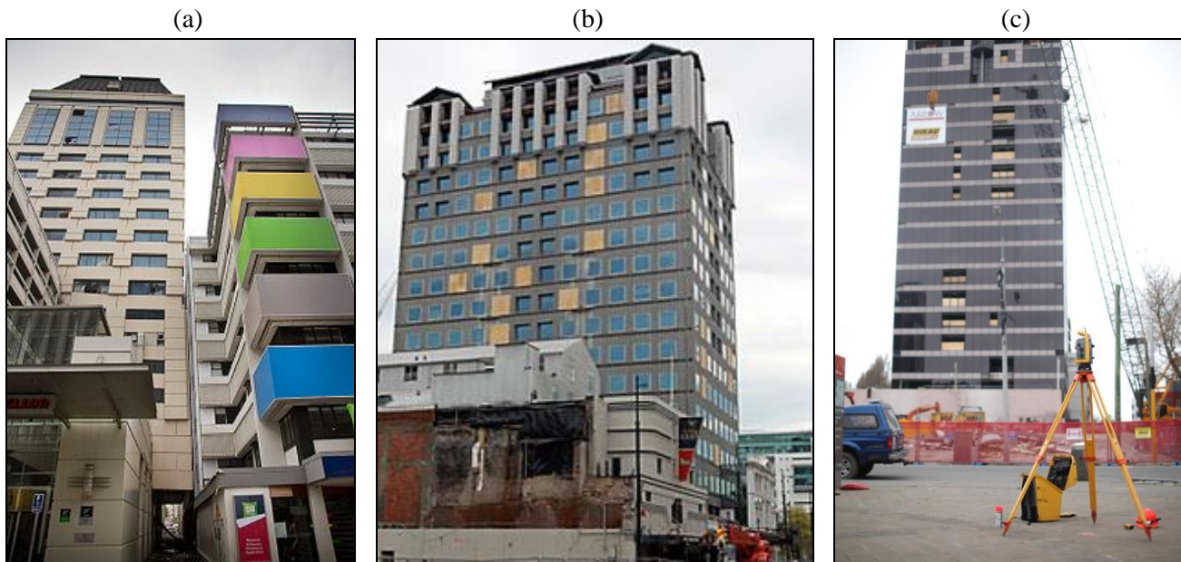
Fig. 3 – Buildings damaged during the 2010 – 2011 Canterbury earthquake sequence that were subsequently demolished: (a) Hotel Grand Chancellor 1 ; (b) Clarendon Tower 2 ; (c) PricewaterhouseCoopers building 3
