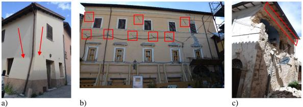
Figure 5: Restraining elements observed in Norcia: a) buttresses, b) ties o c) concrete ring beams Conversely during the site investigation, no buttresses were observed in Amatrice. The main building stocks' characteristics are summarized in Table 2
