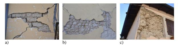
Figure 2: Details of the M1, M2 and M3 masonry types in Norcia
