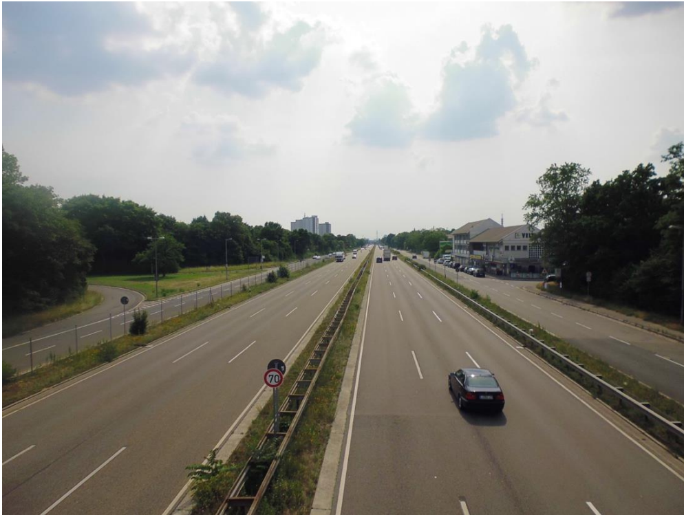
675 Figure 8: The highway B38. BFV is situated on the right.
