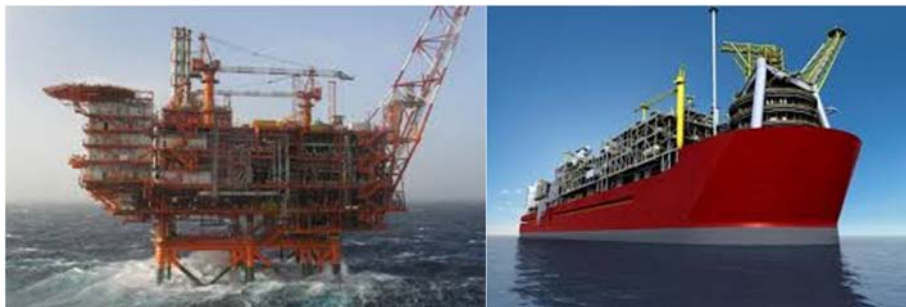
Figure 1. Living quarters of ships and offshore structures made of thin plate panels.
