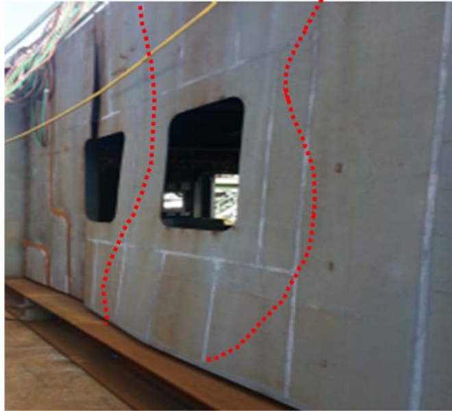
Figure 22. Thermal buckling occurred in thin plate panels with a thickness of 6 mm.
