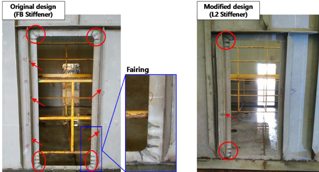
Figure 26. Fairing work of the doorframes to remove the welding-induced deflections for the original versus modified designs of the target plate panel.
