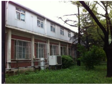
Fig. 2 The case study building
