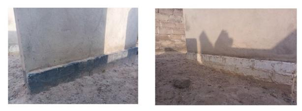
Fig 13b Photographs showing the conditions of the treated walls in the dry season
