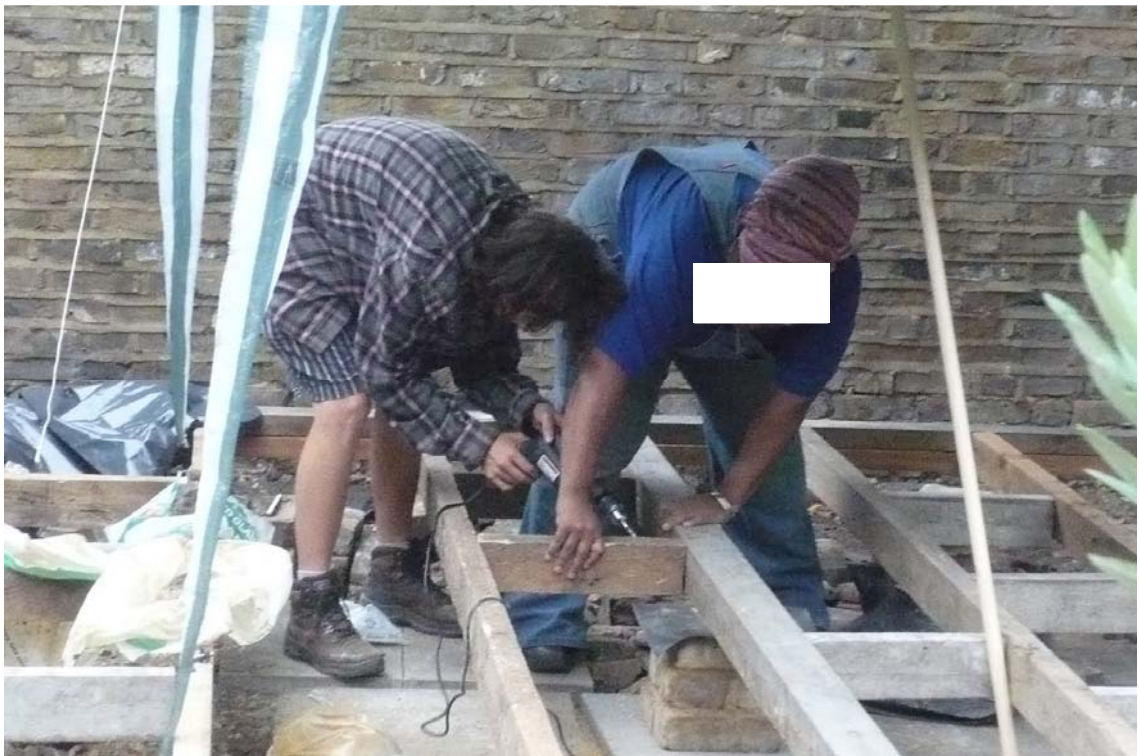
Figure 14: Build day at LCHC pilot site
