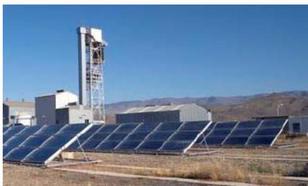
**Figure 2.14** Non-concentrating solar collectors - flat plates at PSA, Spain (source: <http://www.psa.es/webeng/instalaciones/desalacion.php>). PSA: Plataforma Solar de Almería.
