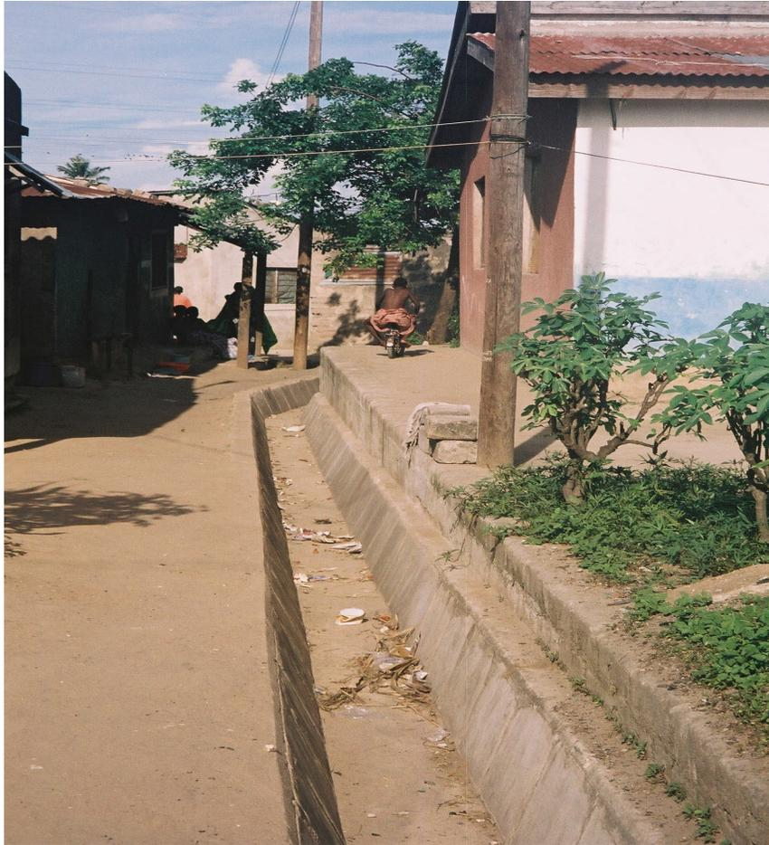
**Figure 13 Well-maintained drainage in Mburahati Barafu**
