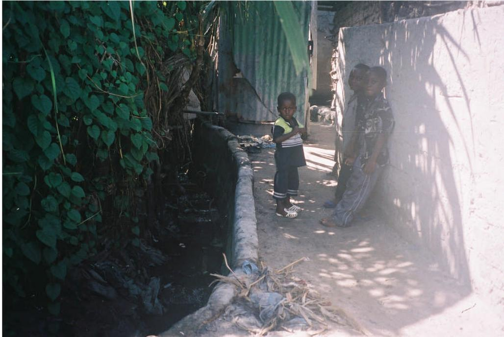
**Figure 16 Self-constructed drainage in Hana Nasif**
