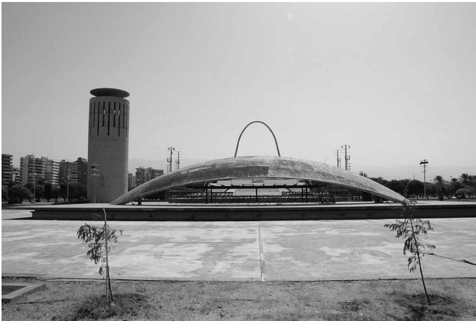
Figure 3. Concert Hall shell. Exemplifying the virtuosity of the engineering and construction in many of the pavilions, the in-situ concrete construction of the shelter covering the concert stage narrows to an impossibly thin 50 mm in its centre (photograph by David Burns).
